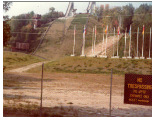
New England Bus Tour, 1982 Ski Lifts in New Hampshire
